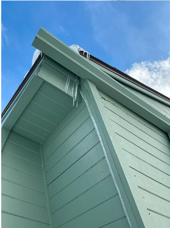
Photos 18-21: Ice buildup and exterior damage at NW corner of building (Anderson Hallas Architects 2025)
