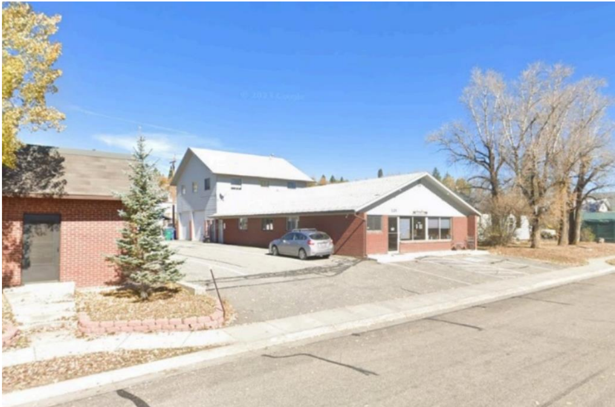
Photo 41: Exterior of District Offices (Google Maps Streetview 2023)
