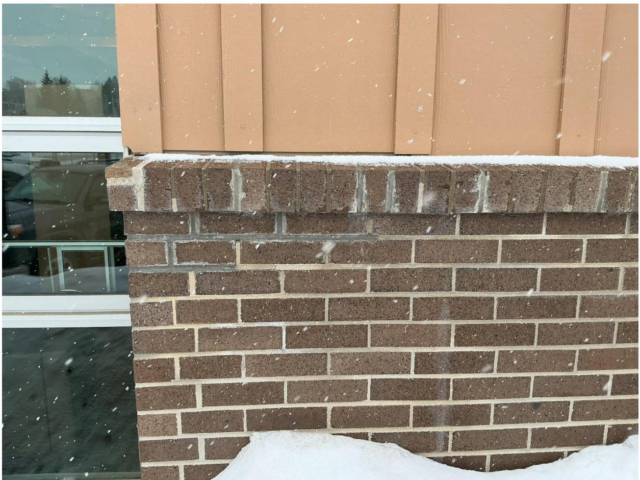
Photo 6: Repaired rowlock ledge. (Anderson Hallas Architects 2025)
