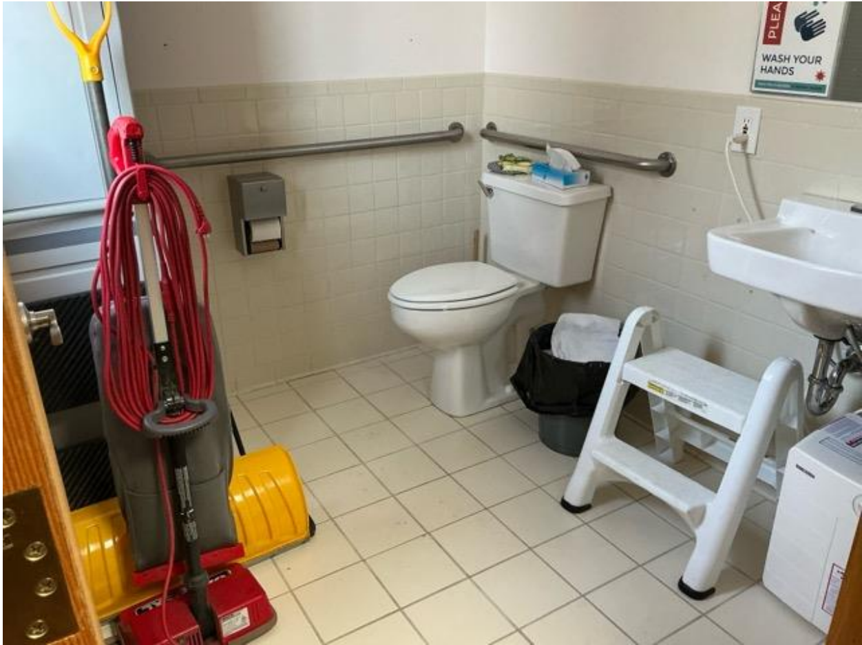
Photo 38: Restroom (Anderson Hallas Architects 2025)
