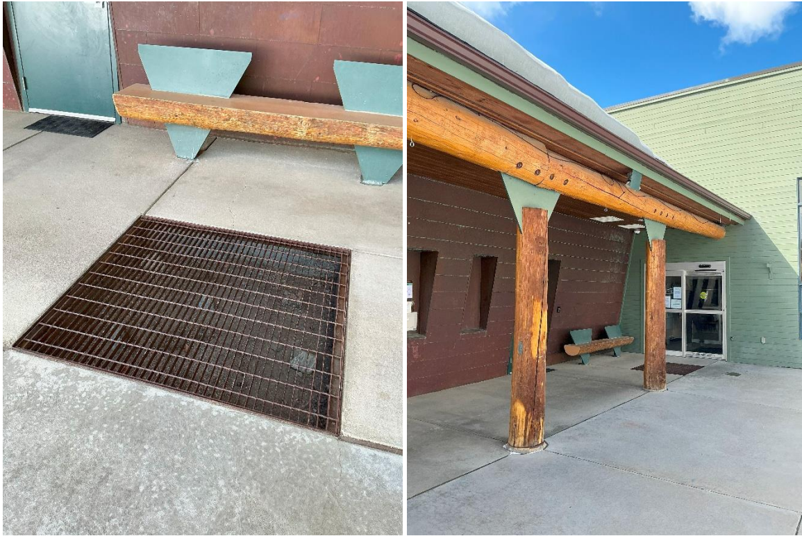
Photo 16-17: Walk-off grate at Library entry (Anderson Hallas Architects 2025)
