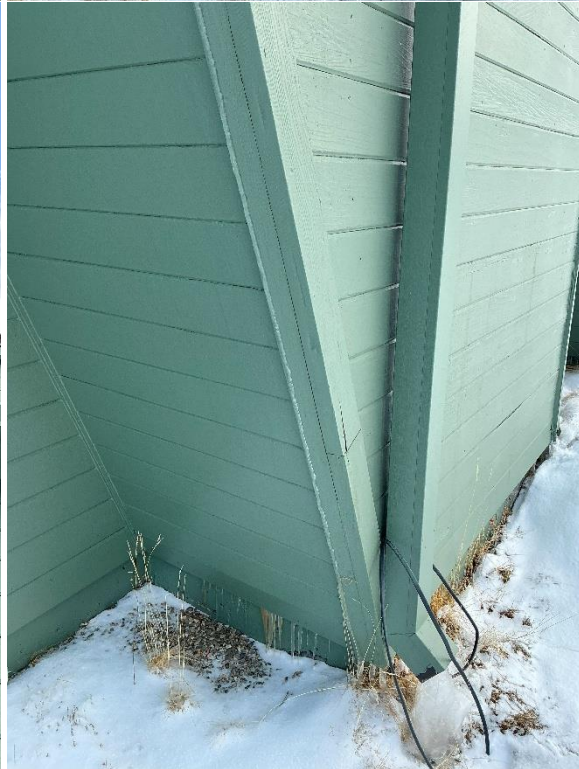
Photos 18-21: Ice buildup and exterior damage at NW corner of building (Anderson Hallas Architects 2025)
