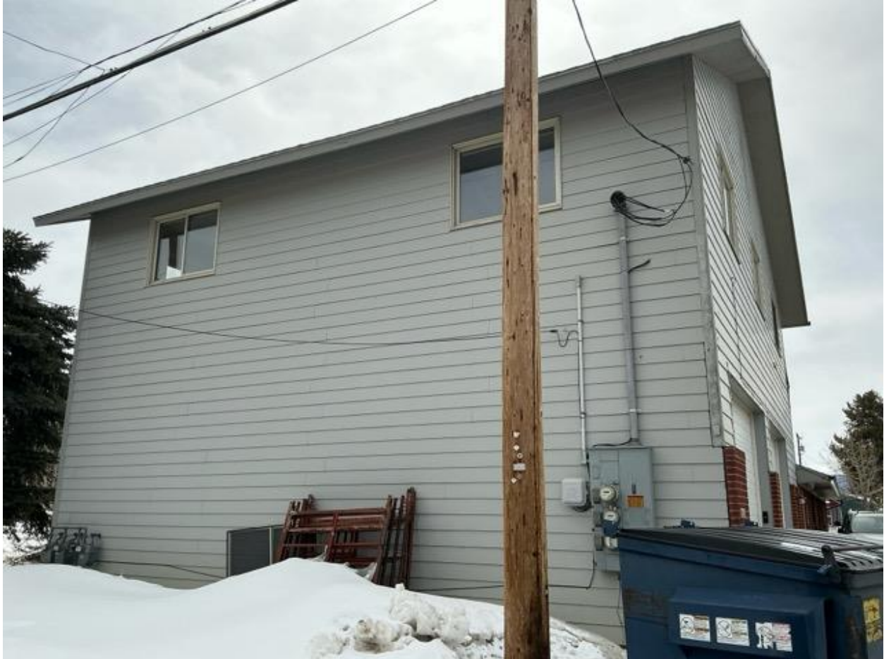
Photo 41: Rear exterior of District Offices (Anderson Hallas Architects 2025)
